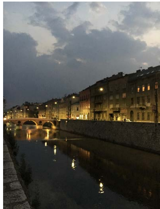
Fig. 4: View of the Latin Bridge in Sarajevo
