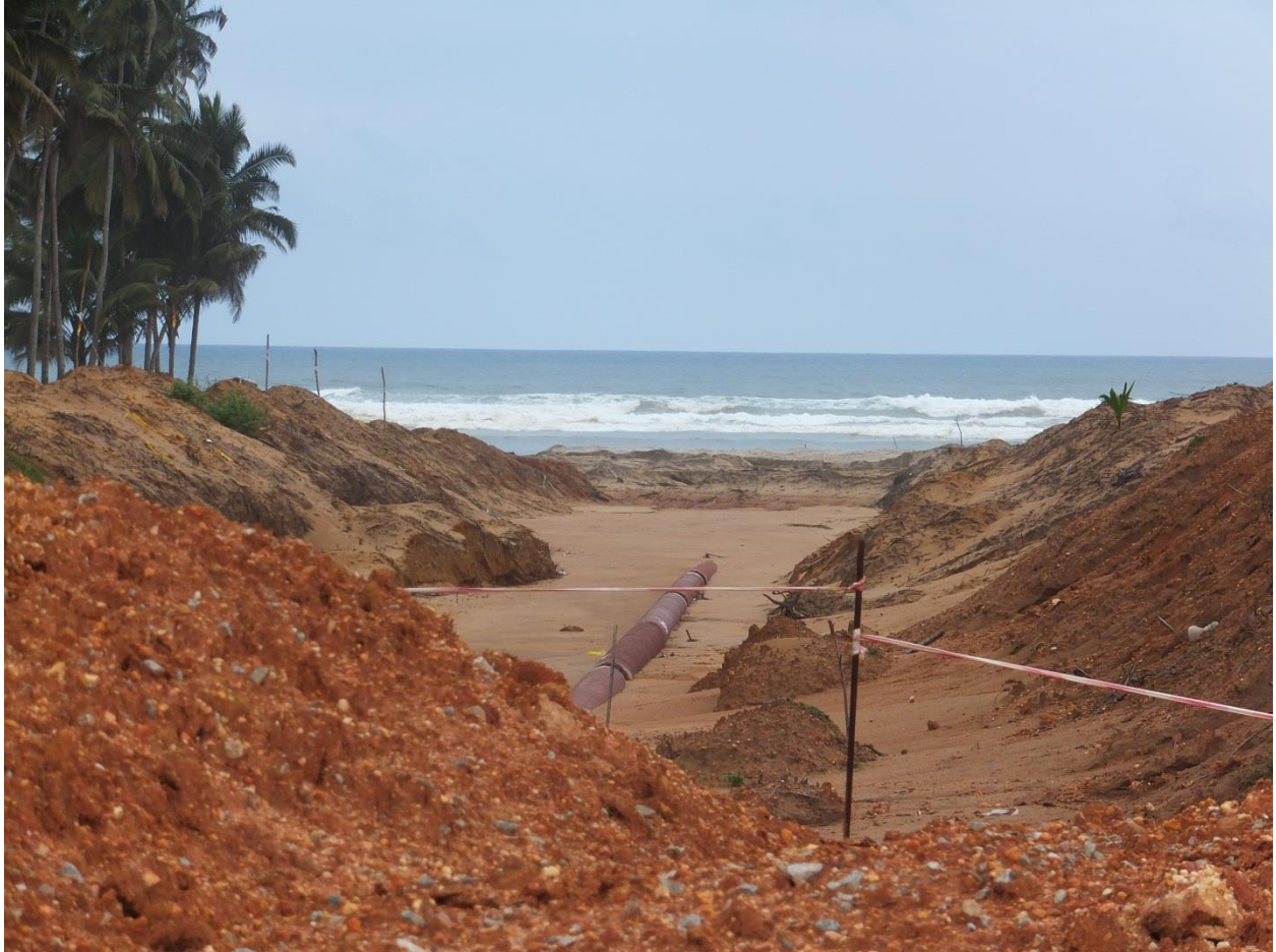
The point where the onshore pipeline begins.
